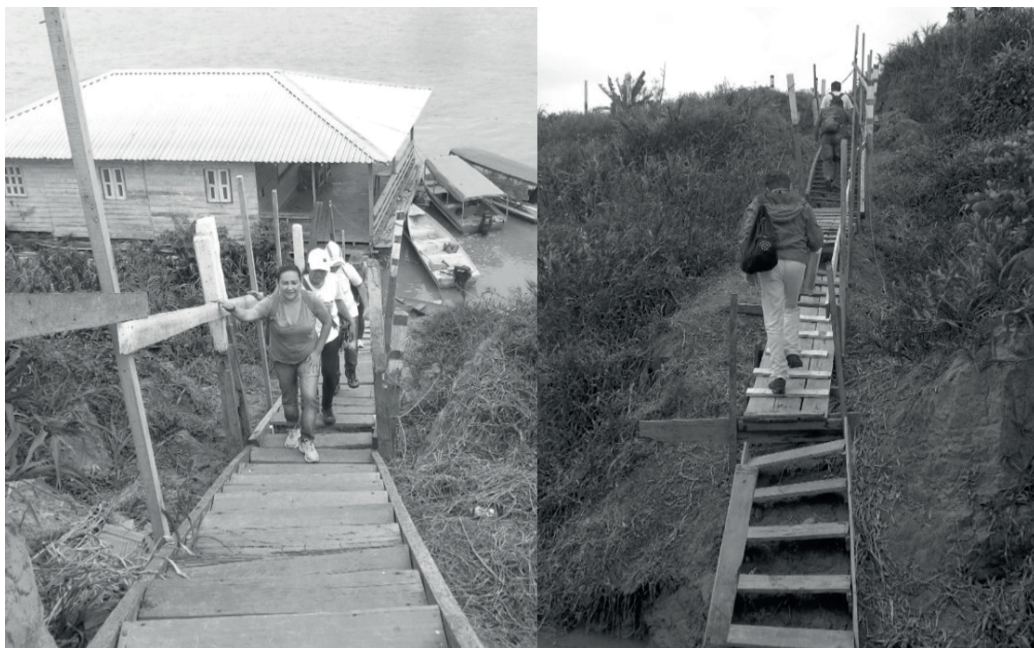
Figure 8. Aspects of unstable (concave) margin of the river channel at Paraná of Terra Nova, called “ barrancos ” (unstable ravines). Up-down view (right) and bottom-up view (left). Source: RESILIDADES project, 2016.
